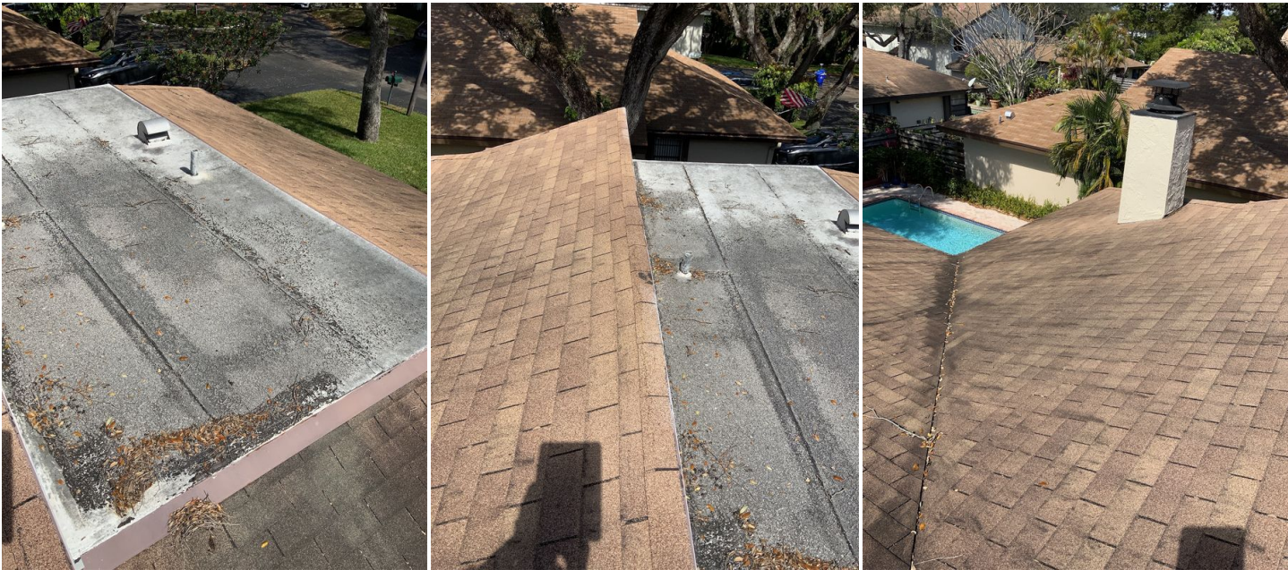
Photos of Each Slope
